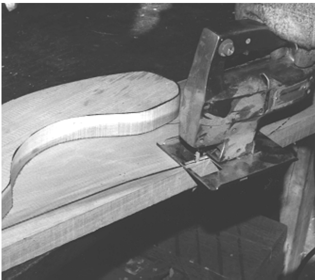
Figure 18: A saber saw can cut the layers for a laminated beam.
